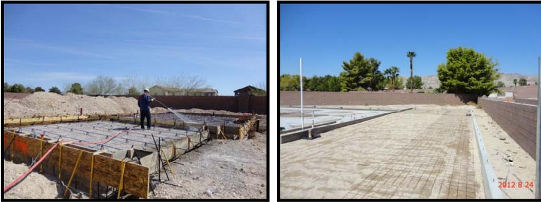
Conventional soil treatments rely on creating a chemical barrier in the soil that is toxic or repellent to termites contacting it. Stem-wall sites, including floating slab sites (left) and monolithic slab sites (right) both require horizontal pre-treatment on the exposed soil surface underlying the structure.
