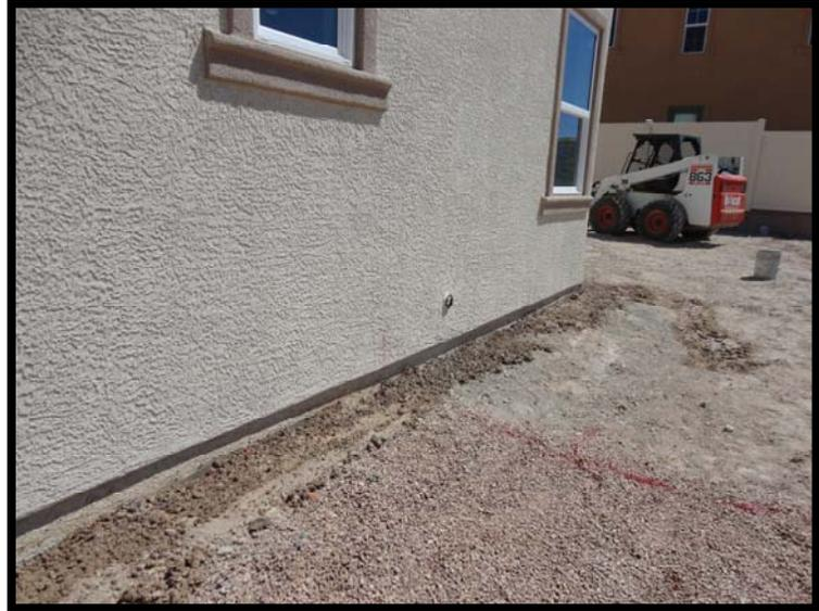
**Termiticide dilution applied to “final grade” trench (left); and treated soil that was replaced into the trench (right).**
